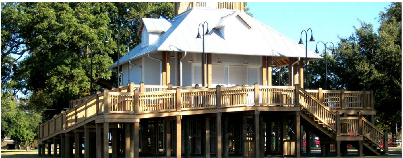
elevated above base flood elevation
